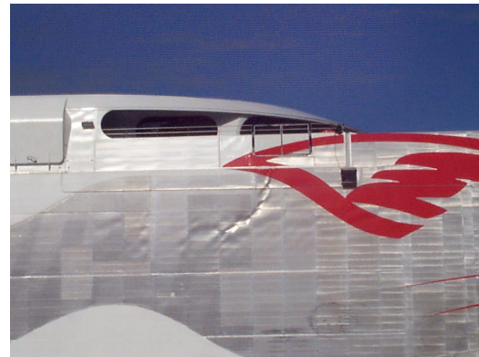
Figure 2: Hull 050 Damage from Extreme Slam Event - External Plating at Frame 51. View showing Buckled External Plating and Sponson
